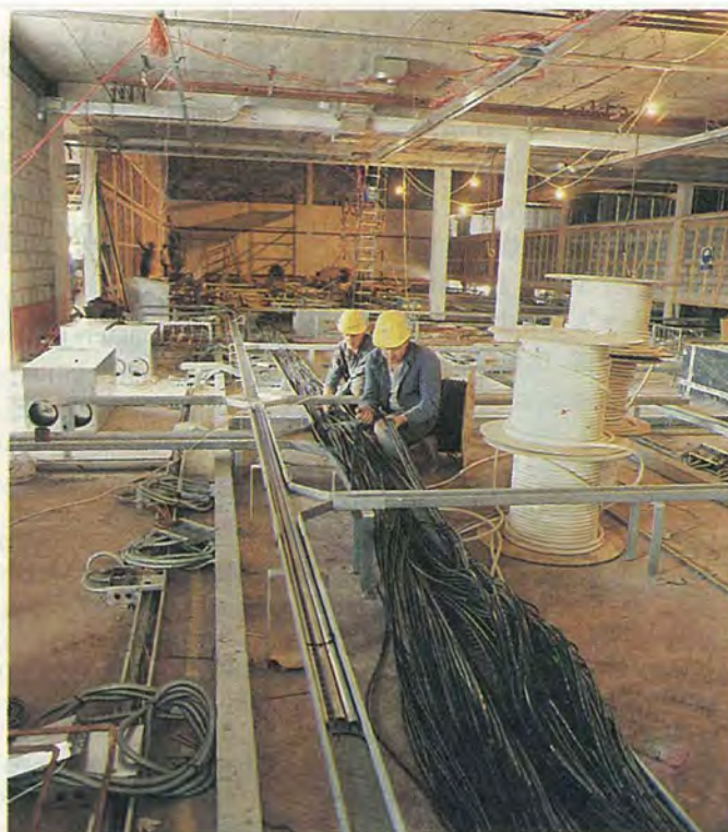
Above: Flashback to the early days and the installation of the underfloor data cabling.
