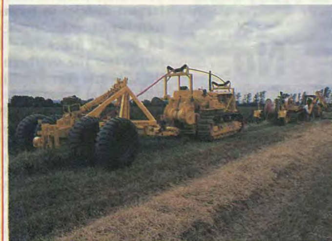
● Ploughing into their work . . . The convoy of tracked vehicles during the high-speed cable laying operation.
